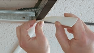
Applying GridMax Over T-bar Suspension Grid System
